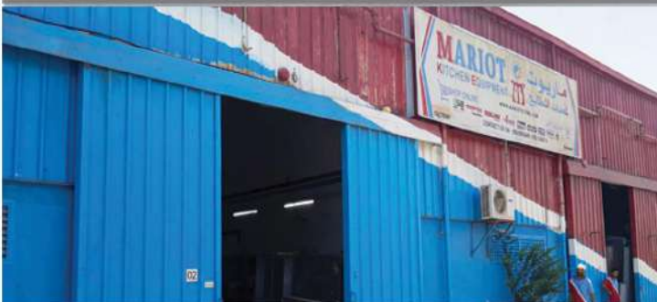
Factory, Industrial Area 11 - Sharjah
